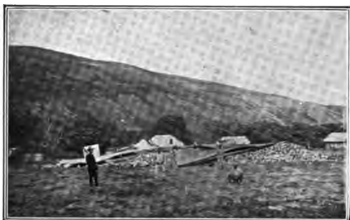
FIG. 68. CHURCH AT WAIOHINU WRECKED BY EARTHQUAKE.
