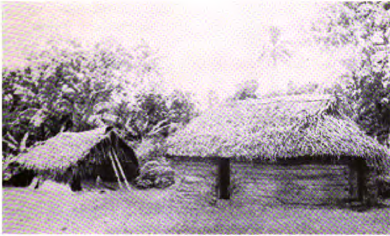
FIGURE 8.—Typical Tongan house showing characteristic oval shape, sugar-cane leaf thatch, and walls of interlaced coconut leaves.
