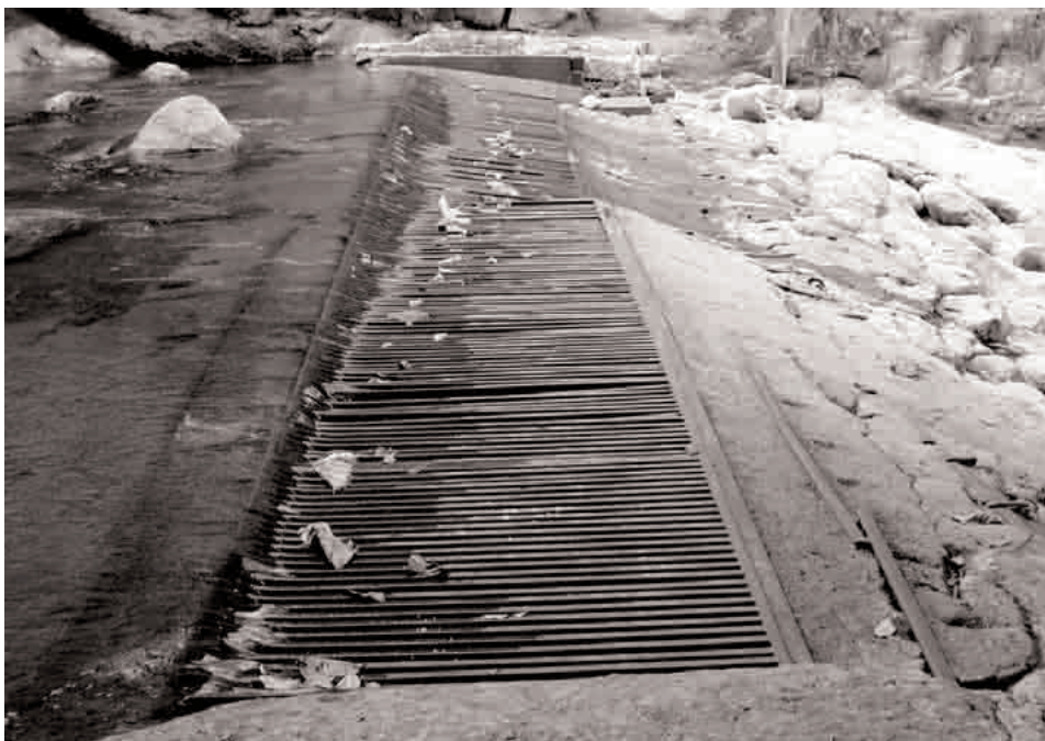
Figure 10. 'Āao Stream Diversion (below USGS Stream Gauge No. 16604500). Most stream flow is diverted into irrigation ditches.
