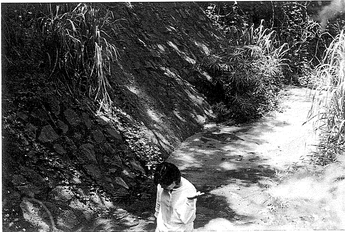
Photo 2. Pool 7, looking makai, showing silty runoff from hydrant flushing (left) down bank into stream
