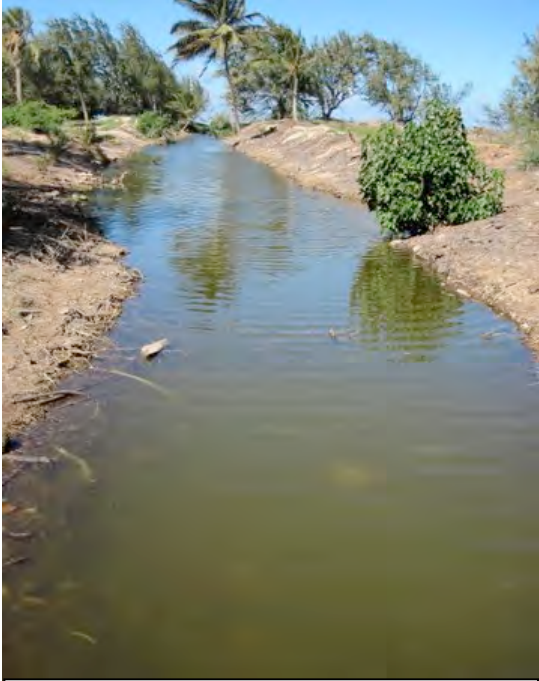
Figure 10. Drainage channel on DLNR property. The makai end in the distance is blocked from the ocean by a sandbar. Photo by C. Imada, HBS.
